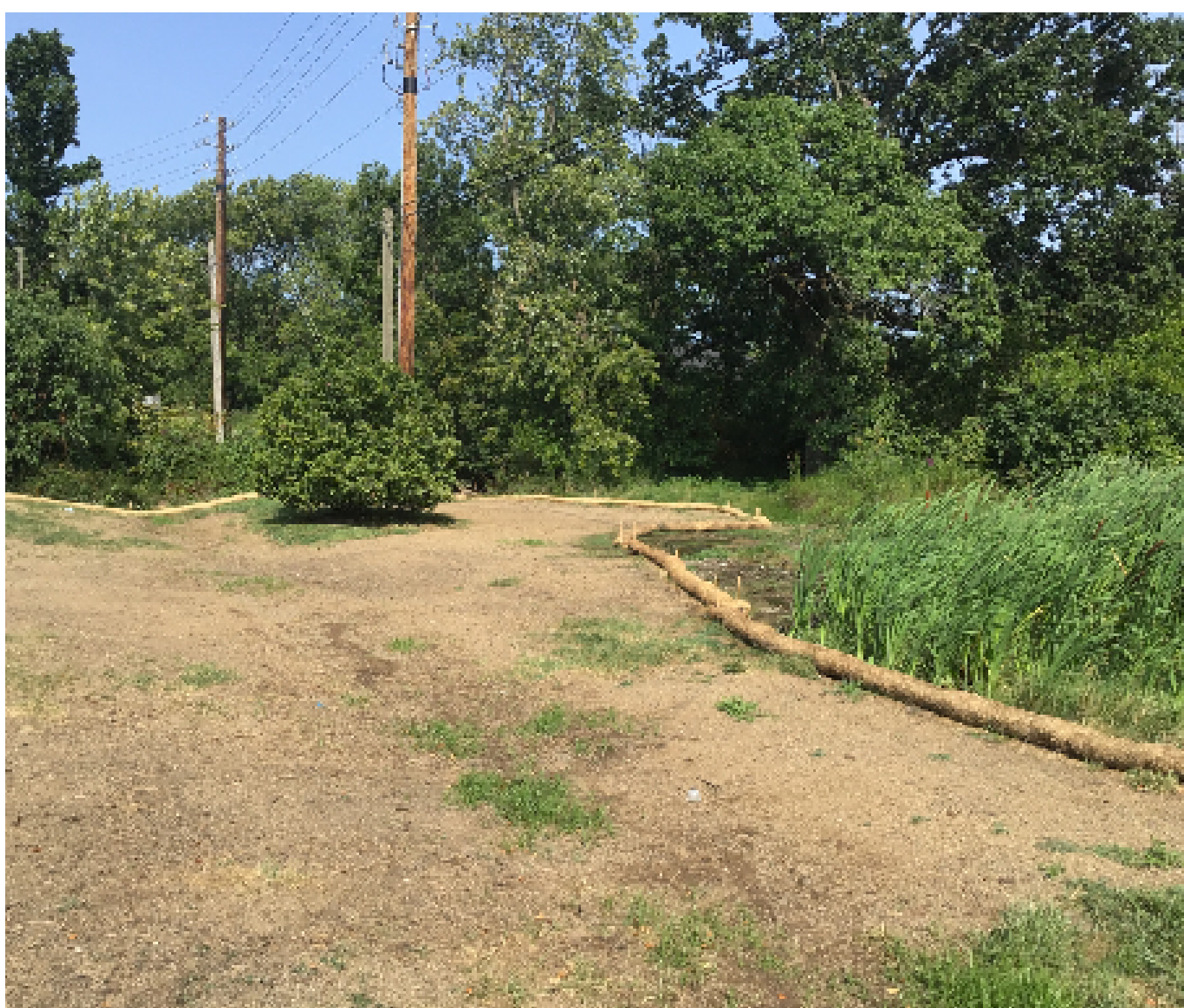
Filter socks stop soil from moving into streams and rivers.
